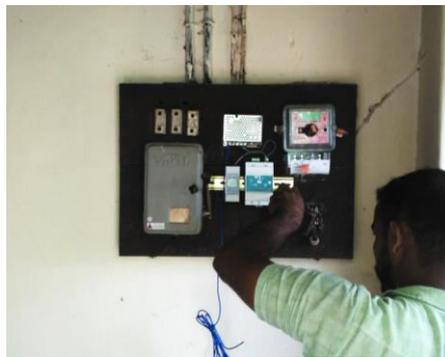
*Data logger: Smart meter and data logger being fixed in a 1BHK home in Kalamassery, South Aluva. The unit measured the consumption every second and logged the parameters into a memory device.*
